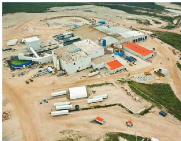
Cameco Corp.'s underground Rabbit Lake uranium mine in the Athabasca Basin about 700 km north of Saskatoon, Saskatchewan. Photo courtesy Cameco Corp.
