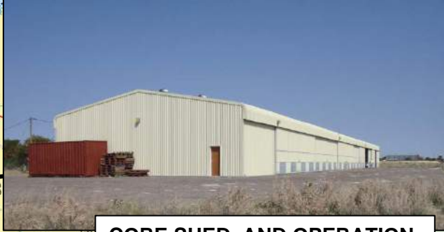
CORE SHED, AND OPERATION FACILITIES, MAUN
